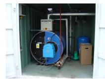
**Boiler upgrades**, upgrade to self monitoring level controls, invertor driven boiler feed pump, modulating feed water, automatic bottom blowdown, TDS blow down controls, heat recovery from blowdown.
